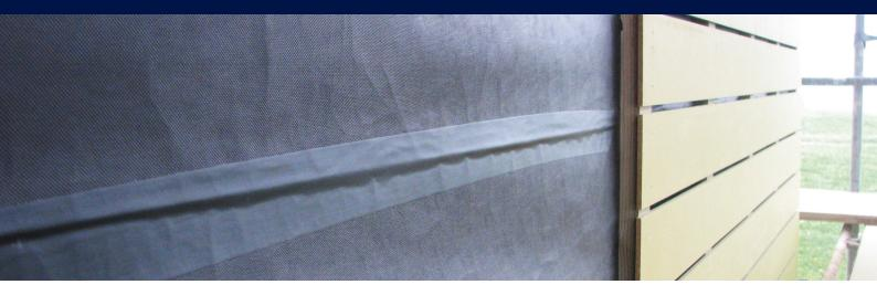
Tyvek<sup>®</sup> Facade tape features a modified water-based acrylic adhesive and a siliconized paper release liner. Tyvek<sup>®</sup> Facade tape has excellent resistance to time, water, moisture, the weather elements and chemicals. Tyvek<sup>®</sup> Facade tape was developed specifically for the Tyvek<sup>®</sup> UV-Facade membrane.
