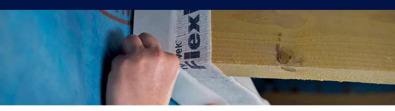
Tyvek® FlexWrap tape is a flexible tape for air and watertight sealing of penetrations at roofs, ceilings and wall. Tyvek® FlexWrap provides an airtight seal and is extremely stretchy compared to standard tape. The unique stretch makes Tyvek® FlexWrap tape easy to fold along deviating penetrations, making it an alternative to standard cuffs. Tyvek® FlexWrap tape is approximately 50% faster to install than standard tape or seals.
