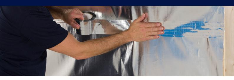
VASTR® Aluminium tape is a single-sided adhesive tape for wind, air, water and vapour tight sealing of overlap seams and repairing damage. VASTR® Aluminium tape is provided with a reinforcement mesh making it very strong.
