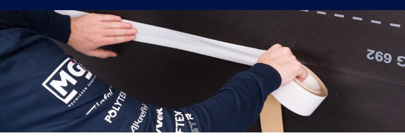
VASTR® Total tape is a single-sided adhesive tape and is universally applicable for membranes and air sealing of the building envelope. The tape in black or white versions features a VASTR® high performance adhesive layer. The top layer of the tape is UV resistant for two years which makes this tape suitable for both indoor and outdoor applications.
